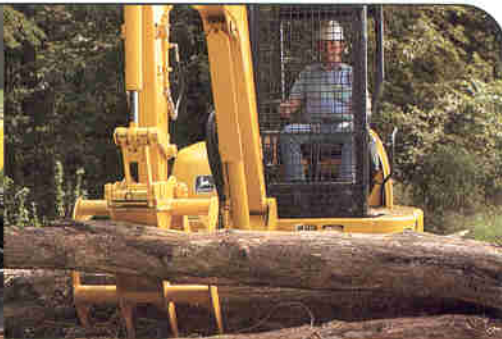
Rake/clamp combo works well for clearing jobs and light demolition work.
