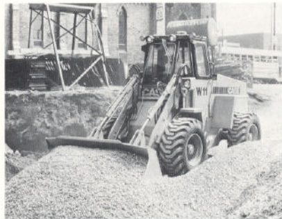
W11 equipped with 1 yd 3 (.76 m 3 ) bucket, cab, 15.00 × 19.5 tires and rear counterweight.
